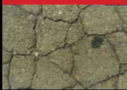
Structurally failed asphalt allows water penetration and contributes to eventual potholes.
