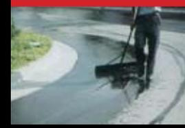
Edgework is most effectively completed using a hand squeegee or broom.
