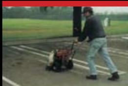
High pressure air blowers and industrial brooms are used to remove surface dirt and debris.
