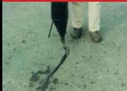
Crack greater than 1/4" width being filled with Western Colloid Flex Crack or hot pour crack filler.
