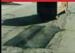
Installation and compaction of hot asphalt to complete repair of damaged area.
